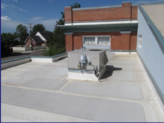
Roof of Addition – Replaced in 2013 (left photo)
